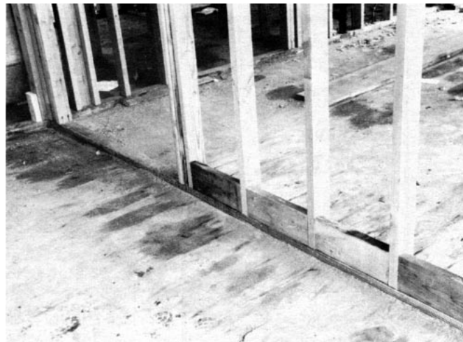
Figure 6. The running 2x6 blocking on the bottom plate provides nailing for the bottom end of wainscot paneling that will sit on top of the baseboard.
