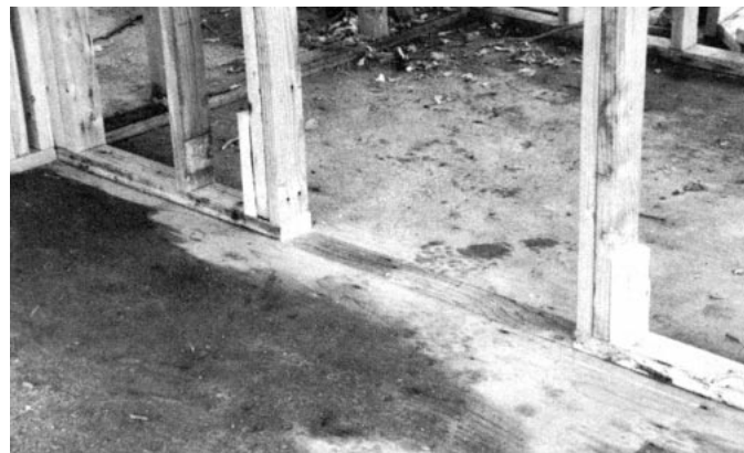
Figure 4. With door casing wider than 2\frac{1}{4} inches, blocking at the base of the door jacks will provide nailing for the baseboard where it meets the casing.
