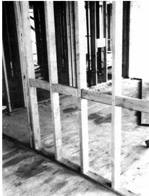
Figure 6. The running 2x6 blocking on the bottom plate provides nailing for the bottom end of wainscot paneling that will sit on top of the baseboard.
