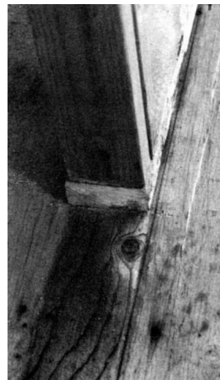
Figure 1. The bottom plate on either side of this rough door opening has been knocked off the chalk line. This will cause problems for the finish carpenter hanging and casing the door.
