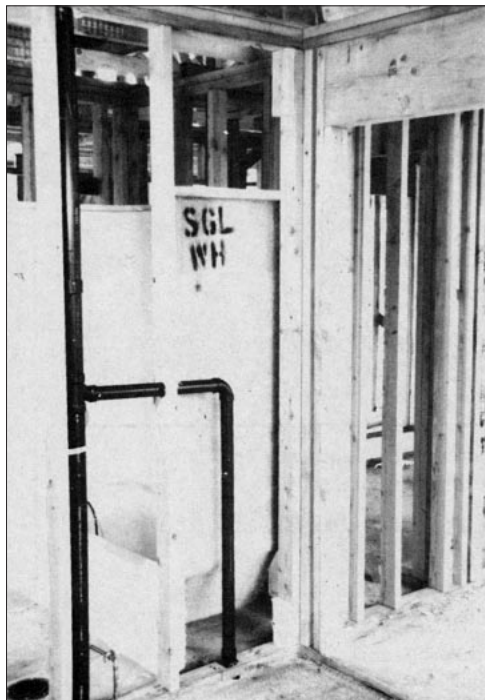
Figure 3. The blocking at the top and bottom of this stud corner will provide good nailing for crown mold and baseboard.
