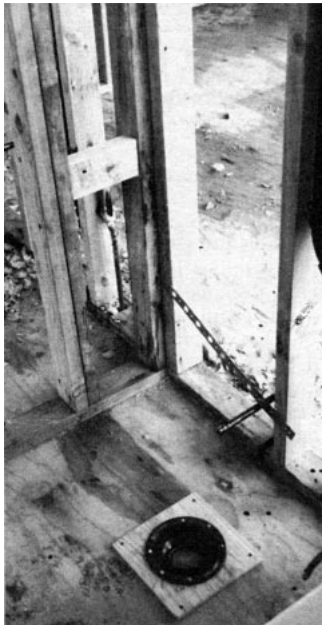
Figure 5. Remember to provide blocking for the toilet paper holder.
