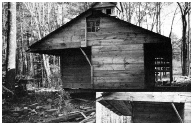
A bearing race from a bulldozer axle became the lazy susan on which the building was turned, using a come-along (operated by the author's wife), while the author (right) acts as human ballast to keep the house level.
