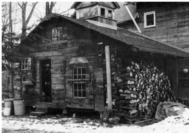
To become a wing of the author's house, this former outbuilding had to be spun 90 degrees and moved 20 feet. The woodpile was added later; but the move was so smooth that several dozen canning jars inside made it intact.
