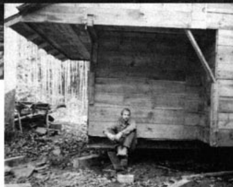
A bearing race from a bulldozer axle became the lazy susan on which the building was turned, using a come-along (operated by the author's wife), while the author (right) acts as human ballast to keep the house level.
