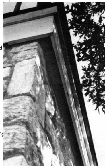
Figure 2. The author detailed the edge of the roof so that water runs off behind the trim boards. The gap behind the trim (above) is hardly noticeable.
