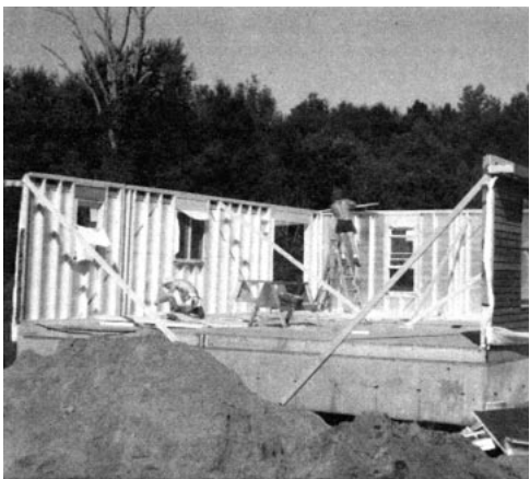
Step 3: A carpenter scabs the top plates to lap at the corners, while another straightens and nails the bottom plate to the deck.
