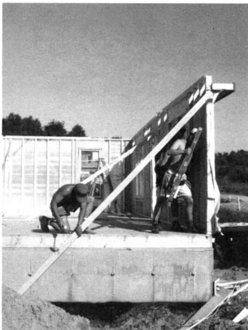
Step 2: After lifting a wall into place, the crew plumbs and braces the corners.
