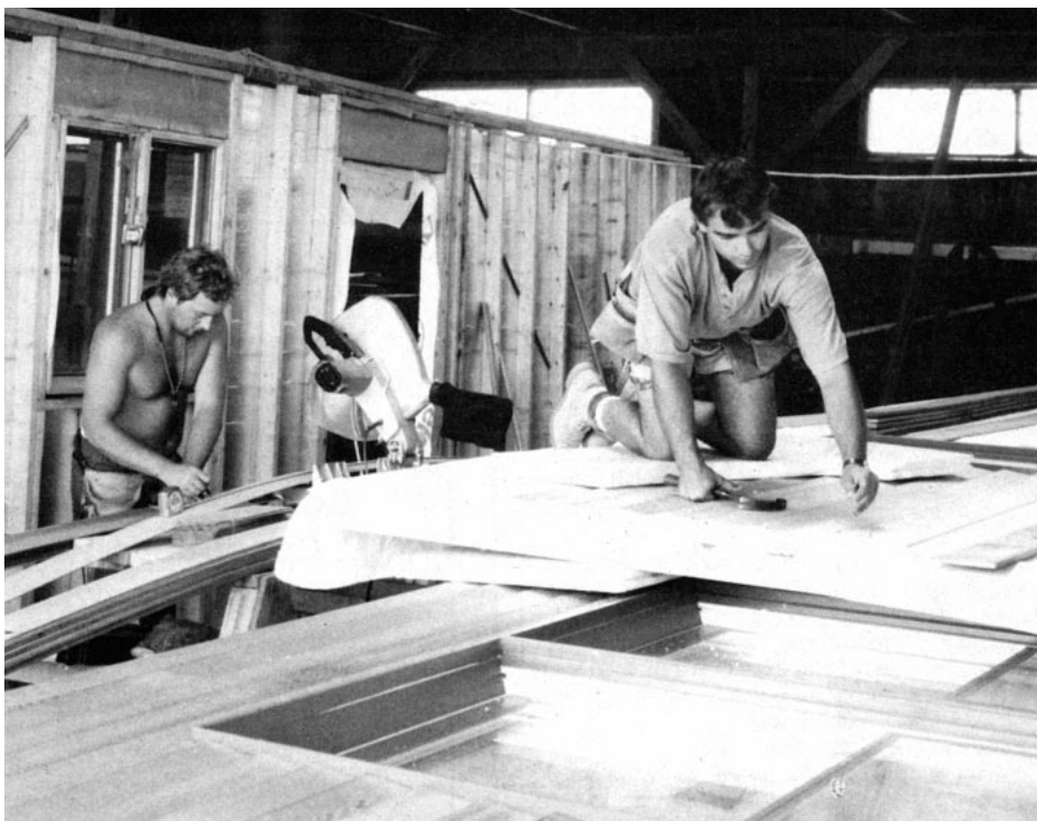
In a converted barn, Hurt's crew frames and sides walls flat on the bed of a house trailer. Above, one carpenter cuts a full bundle of cedar clapboards with a 15-inch chop saw, while another installs the siding over foam sheathing and housewrap.
