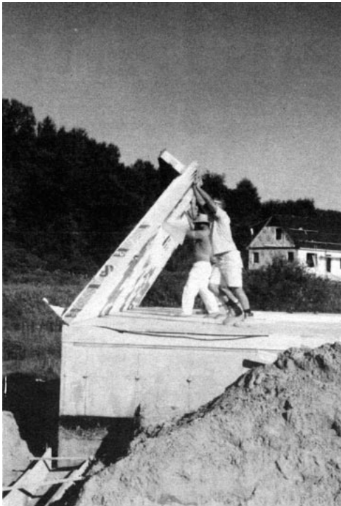
Step 1: Three carpenters can lift a 34-foot 2x4-stud wall sheathed with foam. Lumber strapping is nailed to the bottom plate and to the rim joist to keep the base of the wall from kicking out as it's raised into place.
