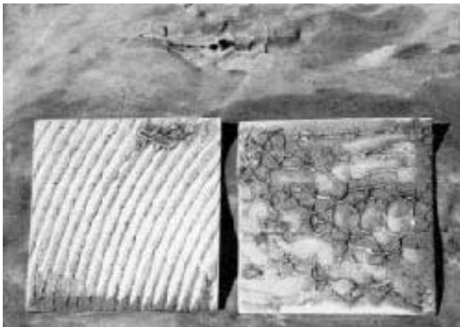
A beating block was used to properly seat the tile on the right, resulting in full coverage of adhesive. The tile on the left was simply positioned and pressed into place.
