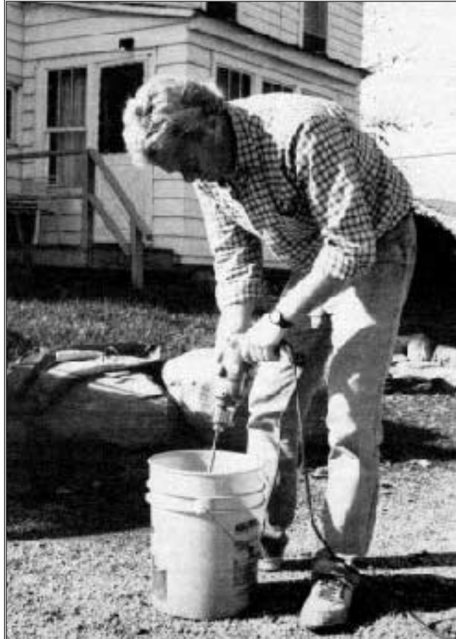
Using a 1/2-inch drill at low speed, the author mixes a batch of grout. Mixing too fast will weaken the grout.
