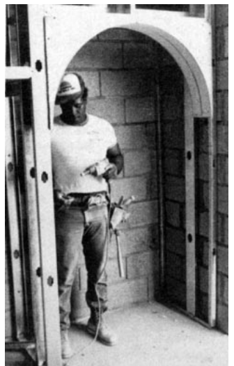
Figure 6. Preformed arch molds greatly simplify framing requirements. The one shown above, from Curvtech , is made of 1/2-inch polyurethane and is covered with drywall paper. Square or bullnose cornerbead are already applied.
