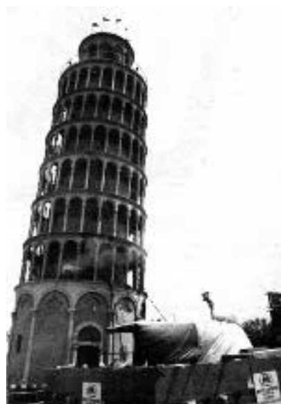
This leaning tower in Niles, Ill., is about half the size of the Pisa original and hides a water tank instead of a bell tower. It is also different in that it doesn't move; the real thing has sunk 7 feet in the last 700 years.
