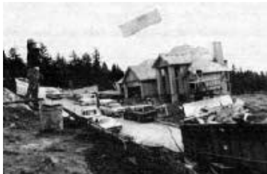
Recycling wood waste is one of the easiest ways to reduce construction's environmental impact. Here a worker tosses waste wood into a clean bin at the 1991 "Street of Dreams" construction site in Tigard, Oregon. He was participating in "Clean Builders," a project sponsored by the Home Builders Association of Metro Portland and Northwest Natural Gas. The project collected and recycled 50 tons of wood, 20 tons of drywall, and 5 tons of cardboard.
