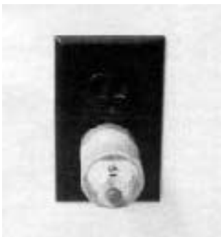
This three-prong outlet looks like it's on a grounded circuit, but using a simple plug-in analyzer the author found there was no ground wire present.
