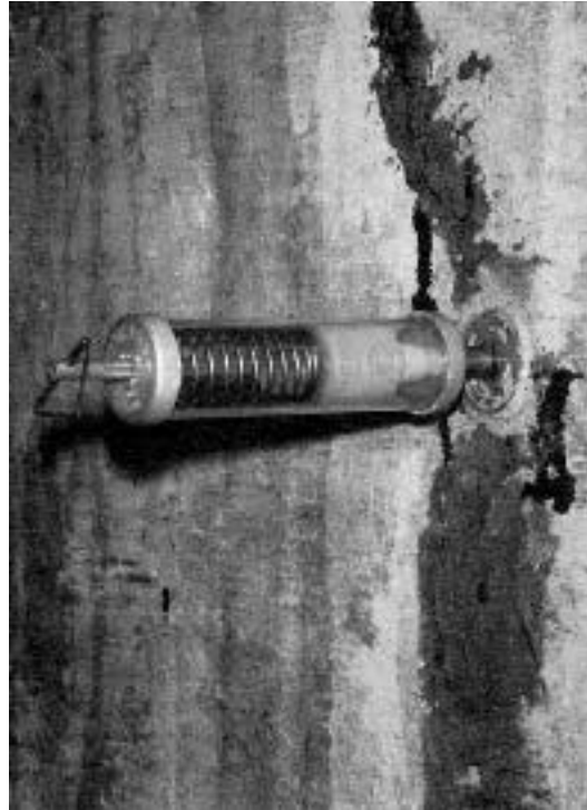
Figure 2. Spring-loaded, low-pressure injection cartridges from Micro Capsule Engineering automatically inject epoxy into hairline cracks, which typically take longer to fill than larger cracks.
