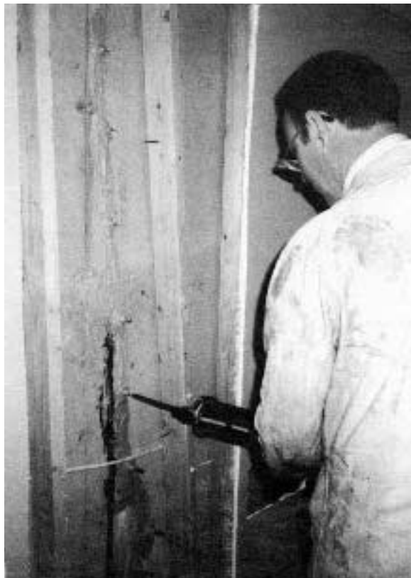
Epoxy is a good choice for repairing leaking foundation cracks. Here, a Jaco contractor installs a flexible epoxy that allows for expansion and contraction.
