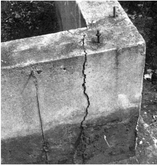
Figure 4. To repair a through-wall crack, like the one in this stem wall (right), first excavate and thoroughly clean the crack. Next, apply the surface-seal epoxy and install the injection ports. Then, working from the bottom port, pump the epoxy into the crack (below) until the material begins to ooze from the port above. As you finish with each port, cap it off and move to the one above.
