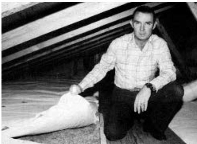
Figure 3. One way to suppress convection in loose-fill fiberglass is to cover the insulation with a convection blanket, such as these pillows manufactured by Attic Seal Inc.
