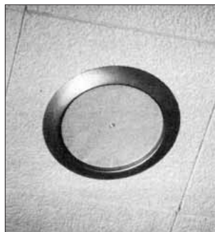
D. Lamps and diffuser are installed.
