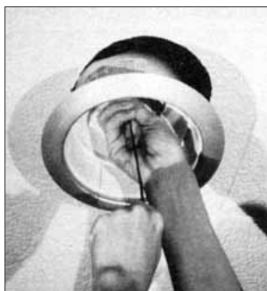
C. The fixture is pulled up against the ceiling using the "zip cord."
