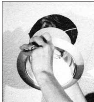
B. The X-18 electrical connector is screwed into the existing bulb socket.
