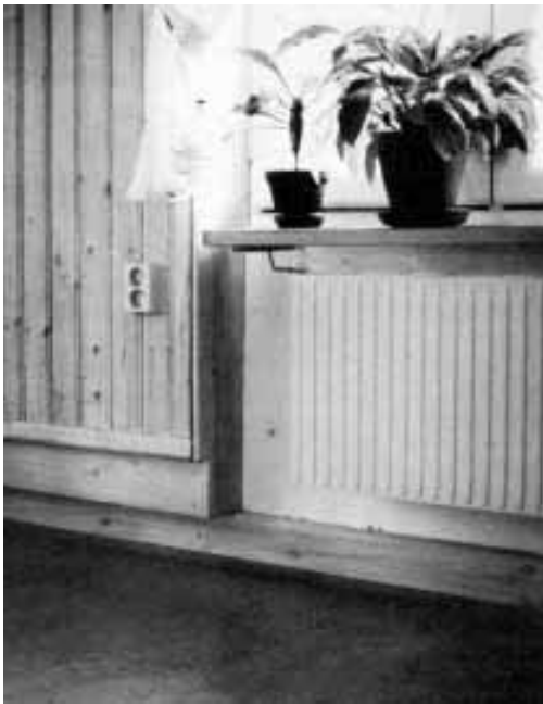
In this experimental Swedish ventilation system, one wall is dedicated to the supply plenum and one to the exhaust. Here, air is exhausted through vents in a kick space on an exterior wall.
