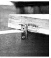
downward pressure on the board to make sure it's tight to the framing, and nail the fastener to the side of the joist. On subsequent courses, repeat the process after first tapping the board into the exposed claws from the previous course. Right- and left-hand versions are useful at butt joints and allow you to conceal the fas-
