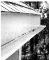
the water away from the fascia and disperse the droplets evenly onto the ground in a 3- to 5-foot band. Available in natural, white, or brown, the sections snap into aluminum brackets that should be screwed to the fascia at least six inches below the edge of the roof. Rainhandler costs about \$4/If and can be ordered from Savetime Corp., 1285 Boston Ave., Bridgeport, CT 06610; 800/942-3004.
