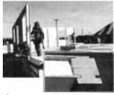
An innovative timber-frame shell package uses premilled timbers and stress-skin panels in a unique configuration that speeds installation, according to the manufacturer. Instead of erecting the wood frame first and then wrapping it with insulated panels, a
