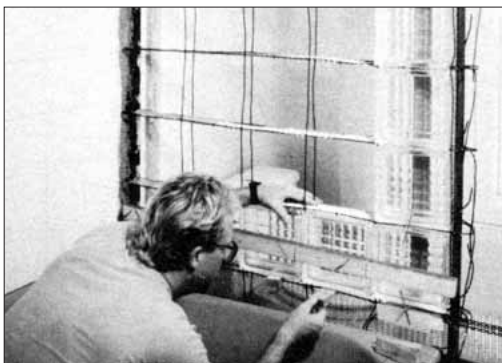
Figure 4. The author places wooden shims to align the courses of blocks as he assembles the wall. He removes the shims after the first application of mortar has set up.
