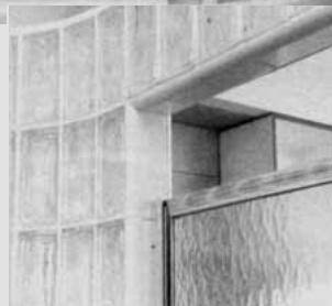
Special fortified mortars have pushed the limits of what is possible with glass blocks. The header above the shower door is supported only by reinforced mortar and trimmed with tile (inset).
