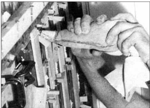
Figure 5. After clamping up a block panel with wooden straightedges — vertical on one side, horizontal on the other — the author uses a heavy-duty pastry bag to squeeze mortar into the joints.
