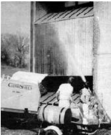
Large painting contractors require a large tank and a heavy-duty airless pump. For smaller operations, rented pumps and small buckets or tanks will suffice.
