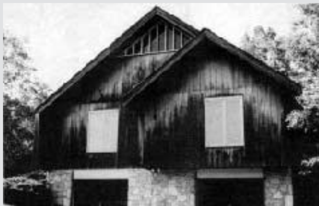
Before: Unfinished siding exposed to sun and rain eventually darkens as the surface degrades, turning gray and providing a habitat for mildew.
