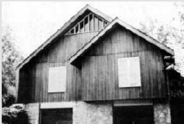
After: Cleaning with a bleach solution, however, can remove the mildew and brighten the wood to close to its original tone. It can then be protected with a clear or tinted finish.
