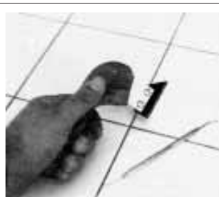
Figure 1. With these tools, and a little elbow grease, cleaning and regrouting tiles becomes an easier task. This little handsaw, from Superior Featherweight Tools, can be used to chip old grout out of tile work. A dental pick, at right, is good for narrow grout lines and corners.
