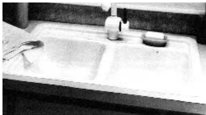
Figure 2. A flush-set sink, like the one in this laminate countertop, takes time to install. But the low-profile sink rim doesn't create a roadblock for sweeping water and kitchen scraps into the sink.
