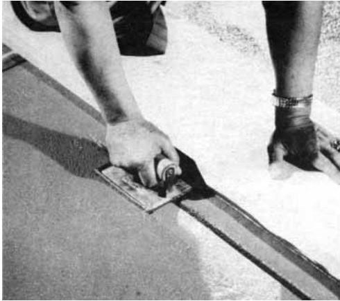
Figure 4. Control joints can be made in wet concrete with a jointing trowel (left) or by forcing a preformed joint material into the surface. In concrete that has already set, you can cut control joints with a concrete saw (right). All control joints should penetrate into the slab at least one quarter of its total thickness.
