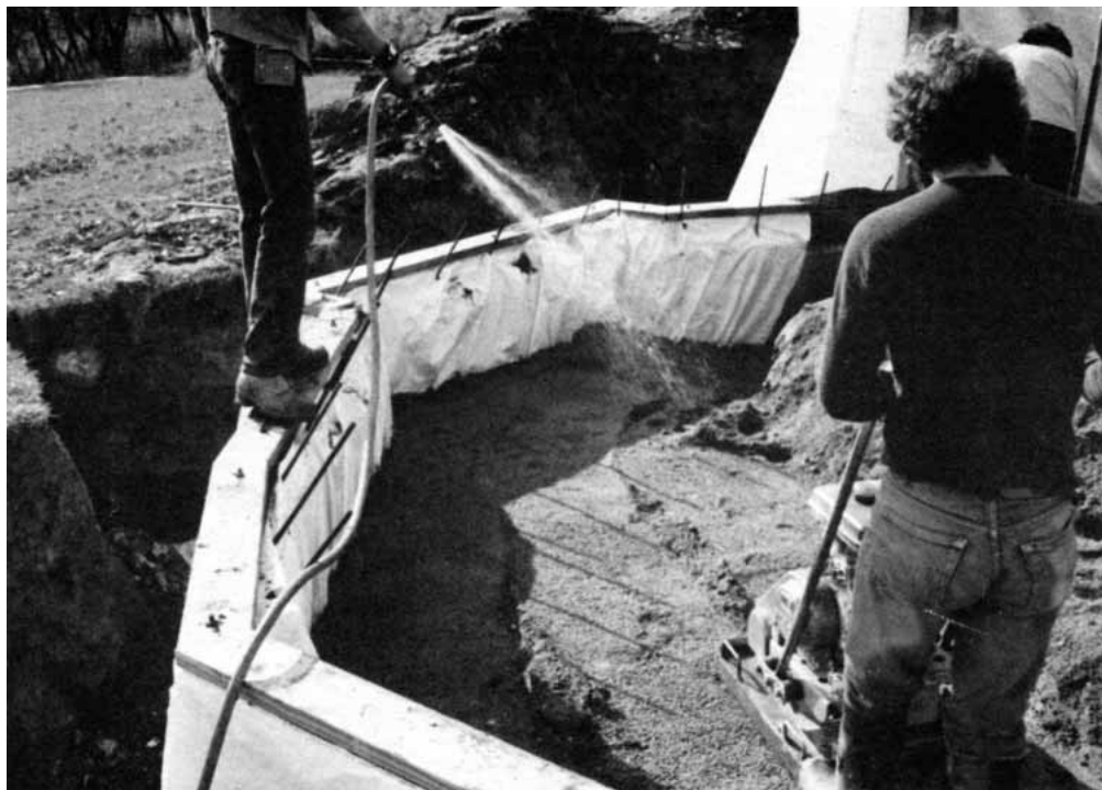
Figure 2. For good compaction, run a plate compactor uniformly over granular fill. Each fill layer should be no thicker than 6 to 8 inches. If the fill is too dry, spray it with water, but avoid puddling.
