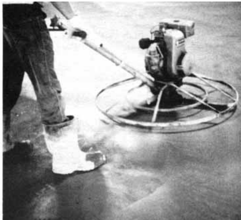
Figure 5. A darby is used to smooth the surface of concrete that is still wet (left). A power trowel, at right, greatly speeds finishing, even on small slabs. Most floor masons carry a spare because there is nothing more nerve-wracking than trying to repair a floor machine while you watch the slab set.
