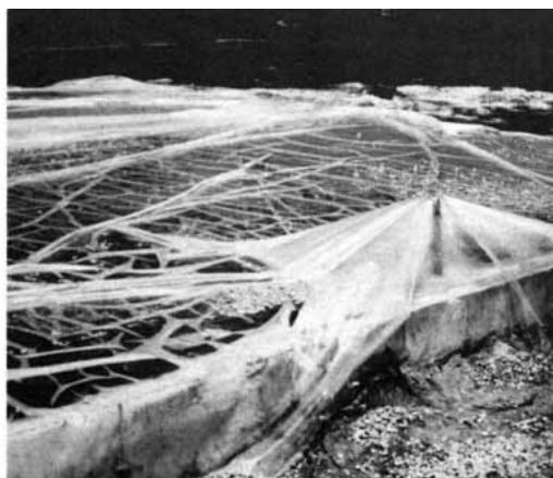
Figure 6. To keep a slab from drying too fast, cure for at least seven days by coating it with a curing compound (left) or covering it with poly sheeting to help hold in the moisture (right). You may need to sprinkle a curing slab with water to keep the temperature below 70°F. In cold climates, heat the slab indirectly to keep it above 40°F.
