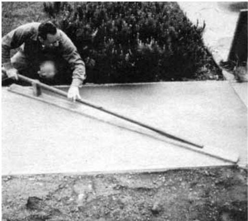
Figure 5. A darby is used to smooth the surface of concrete that is still wet (left). A power trowel, at right, greatly speeds finishing, even on small slabs. Most floor masons carry a spare because there is nothing more nerve-wracking than trying to repair a floor machine while you watch the slab set.
