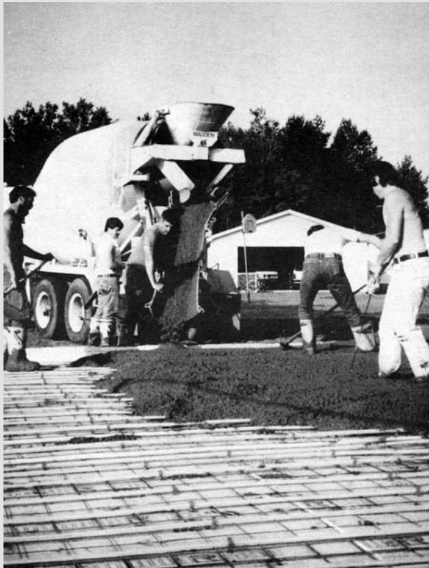
During the pour, at least one mason, shown far right, is assigned the sole task of lifting the welded-wire mesh to make sure the reinforcement and the hydronic tubing end up in the center of the slab section.
