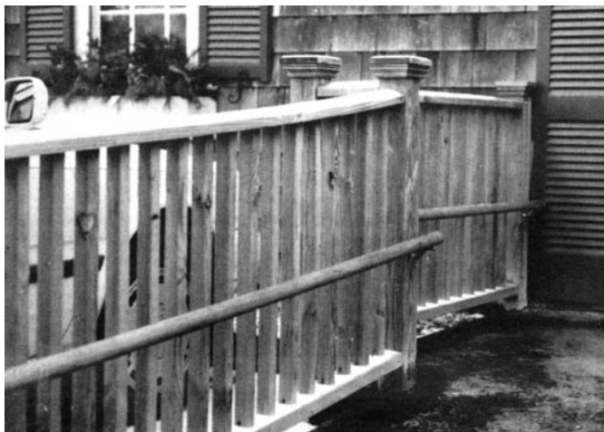
Figure 2. A second handrail installed at a lower height makes it easier for those in wheelchairs to pull themselves up an access ramp. For wheelchair use, the slope of a ramp should not exceed one in twelve.
