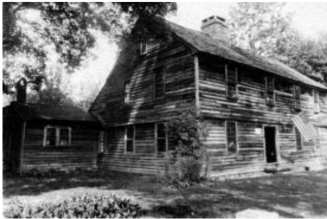
It took ingenuity and a modern sprinkler system to bring the 300-year-old Deacon John Grave House in line with current Connecticut codes.
