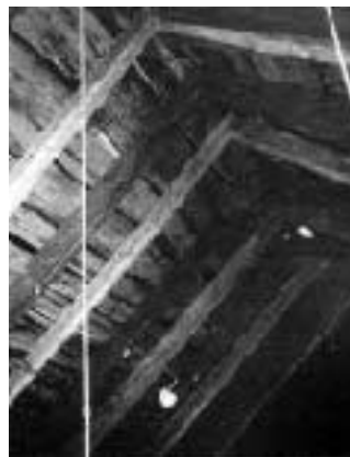
To beef up the roof system, the renovation crew added steel tension rods and new rafters between the old ones.
