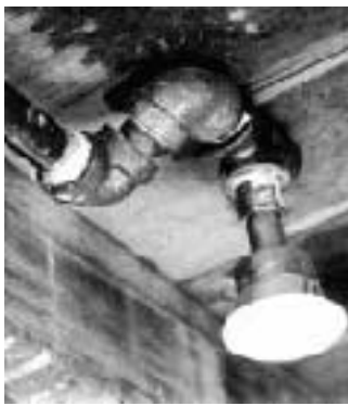
Installing a commercial-duty sprinkler system persuaded the fire marshal to grant approval for the restoration.
