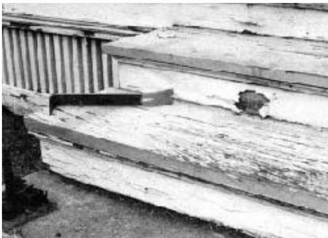
Figure 1. Paint peeling down to bare wood indicates excessive moisture in the woodwork. The buckling paint on the second riser is a result of decay.
