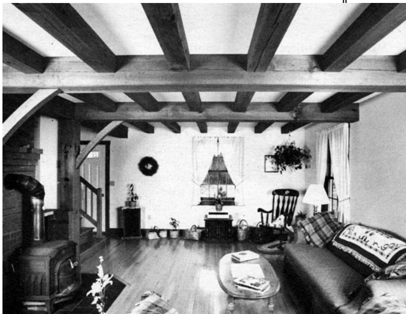
A traditional timber-frame ceiling and 8x8 posts adorn the “great room” of an otherwise conventionally-framed house.
