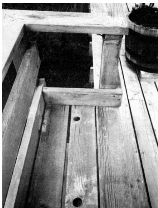
Figure 3. On a stained deck it's hard to tell if the wood has suffered moisture damage, because the stain doesn't peel noticeably. This deck (left) looked okay to the homeowner until the day someone stepped through a rotten board. Paint, on the other hand, peels visibly when it is failing to offer protection (above).
