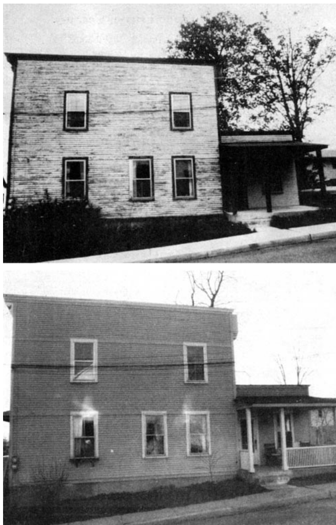
Figure 1. An old house is a good candidate for an alkyd primer and a latex topcoat. The painter scraped the loose paint from this house in Burlington, Vt., (top), then power-washed the surface before coating it with an alkyd primer and two coats of a 100% acrylic paint. The result (above), shown five years later, has yet to show any signs of peeling.
