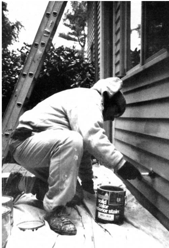
A stain, such as the opaque oil-based product applied here, will need to be recoated sooner than a paint on smooth clapboards. Stains work best on rough-sawn siding.
