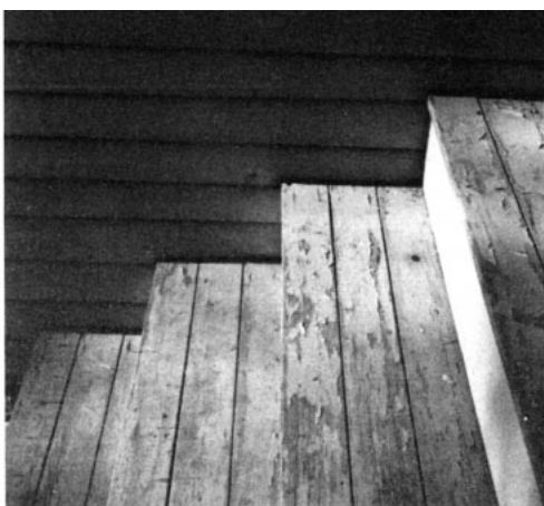
Figure 3. On a stained deck it's hard to tell if the wood has suffered moisture damage, because the stain doesn't peel noticeably. This deck (left) looked okay to the homeowner until the day someone stepped through a rotten board. Paint, on the other hand, peels visibly when it is failing to offer protection (above).
