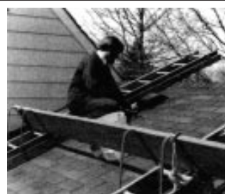
The Ladder-Brace makes a simple-to-use ladder jack for repair work on a pitched roof.
