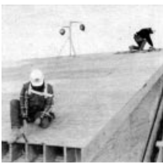
Figure 3. A Whirlie-Bird is the closest thing to a sky hook available for fall protection. The stand, which holds two retractable line reels, must be anchored to the roof with J-bolts that slip through holes in the deck and hook under the roof framing.
