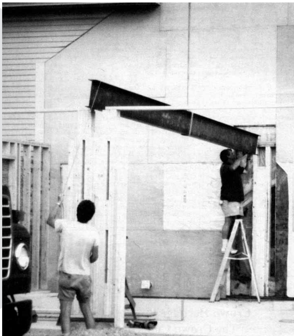
To avoid unnecessary exposure to bad weather, open up only as much of the existing structure as you need to install new structural members, like this steel beam.
