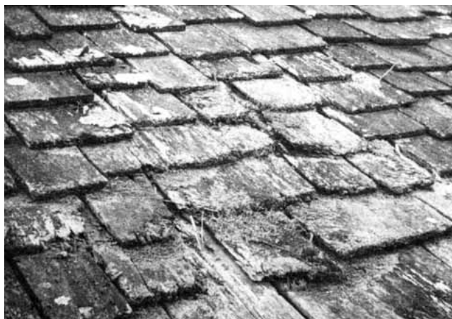
Figure 3. Moss, lichen, fungus, and rot are major enemies of wood shakes, especially where trees overhang a low-pitched roof (above). Periodic cleaning with a power washer (right) can dramatically extend a wooden roof's life span.
