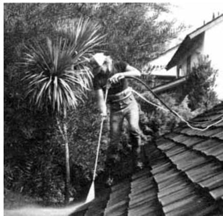
Figure 3. Moss, lichen, fungus, and rot are major enemies of wood shakes, especially where trees overhang a low-pitched roof (above). Periodic cleaning with a power washer (right) can dramatically extend a wooden roof's life span.
