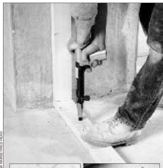
Figure 4. Powder actuated fasteners. For furring out a wall or other light-duty work, PAFs are often the fastest, most economical choice. Current models are much safer than older high-velocity drivers, but safety is still a big concern. A variety of pins is available for different applications (insets).
