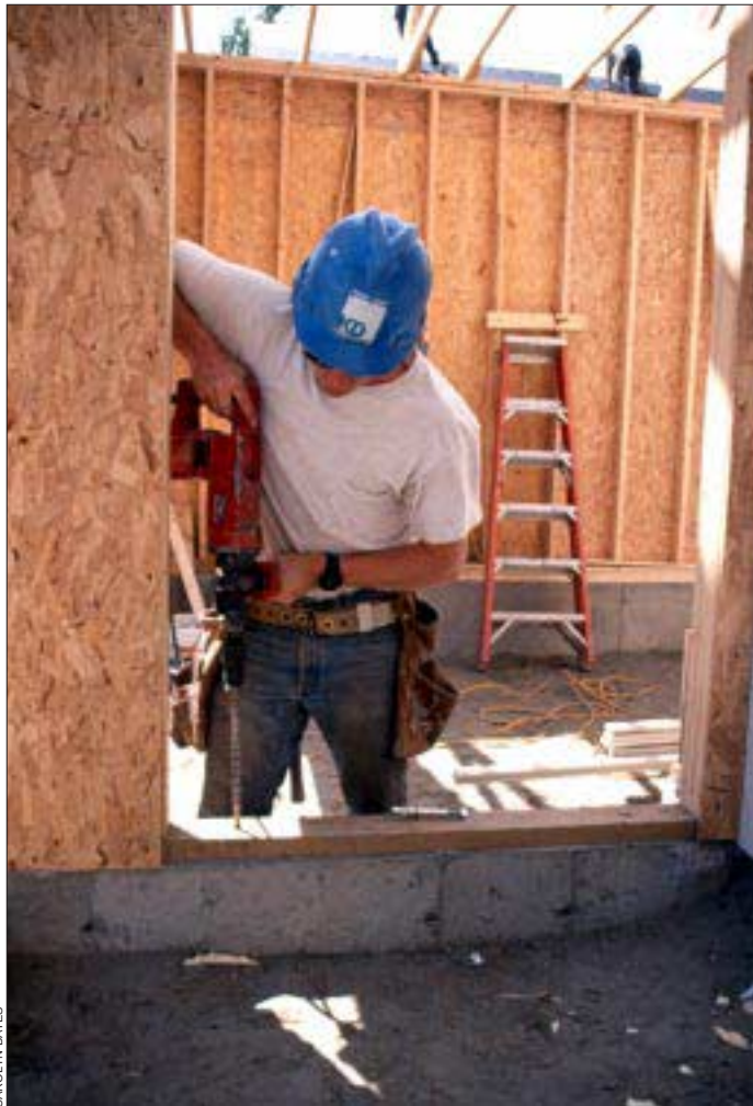
A carpenter drills through a bottom plate into a concrete stemwall to install a wedge anchor — a fastener strong enough to serve as an anchor bolt.
