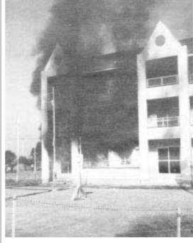
Despite an impressive amount of smoke, the fire did not spread from the first to the second floor until after 72 minutes, when firefighters cut holes between the two floors.
