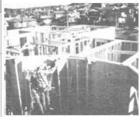
To convince Japanese code officials that three-story wood-frame construction can stand up to earthquake and fire, the American Plywood Association built a mockup of a large multi-unit project — just so it could be shaken and burned.
