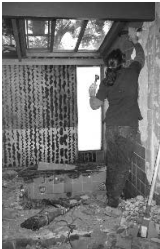
Figure 2. A worker removes ceramic tile from a crumbling green-board substrate in a tiled whirlpool bath. The failed substrate will be replaced with cement backerboard.
