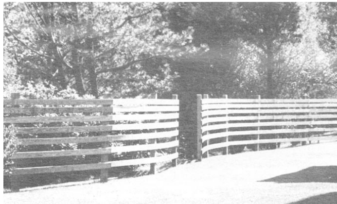
Figure 1. To shelter a seaside garden from wind, the author built this curved frame. The curves serve no wind-breaking function; the secret to the fence's wind-cutting ability is in the graduated spacing between courses.
