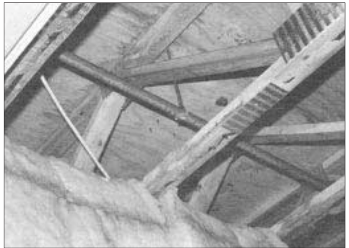
Drip-marked pipes and stained insulation indicated too much moisture in the truss floor cavity.
