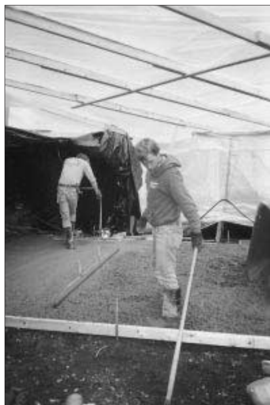
Figure 4. In order to pour sidewalks in sub-freezing weather, these concrete subs erected a temporary plastic tent and supplied heat with a salamander heater.
