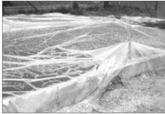
Figure 1. Polyethylene film will prevent moisture from escaping from wet concrete in warm or windy weather, but it may discolor the concrete where it comes in contact.
