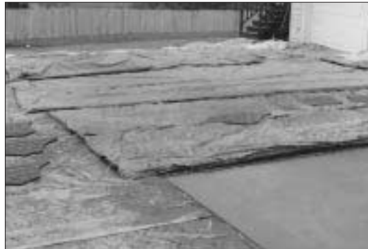
Figure 3. In moderately cold weather, insulating blankets can keep fresh concrete from freezing by retaining the heat of hydration.
