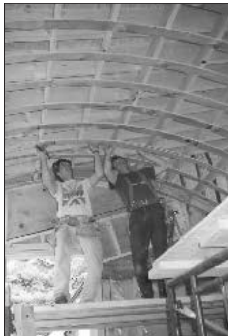
The author, at left, and carpenter John Crosswaithe install a double layer of \frac{3}{8} -inch plywood strapping to the bottom of the barrel vault's 2x8 joists.
