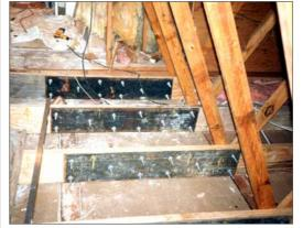
Ten Micro-Lams, spliced together with 48-inch-long steel plates, make up five 21-foot floor joists inside the attic. The author drilled the splice plates in an X pattern to fit five 1/2-inch carriage bolts on each side of the splice.
