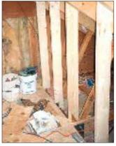
New 2x8 rafters sistered to the top chords stabilize the modified trusses. Two-by-six studs carry the roof loads to the Micro-Lam joists.
