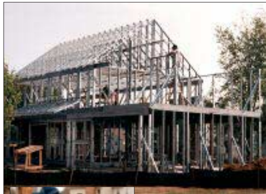
Steel framing got a vote of confidence when NAHB recently chose metal studs for its Resource Conservation House in Bowie, Md. How steel compares environmentally to wood is still hotly debated.
