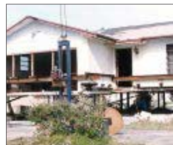
Need a lift? Using a grid of steel beams punched through the walls, LiftPlate International raises homes — slab and all — for rebuilding safely above the flood plain.
