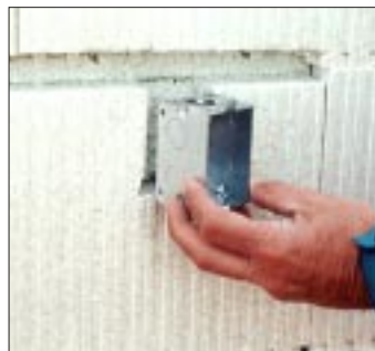
Figure 6. Chasing electrical wires and installing boxes in foam is easy with a router or a hot knife.
