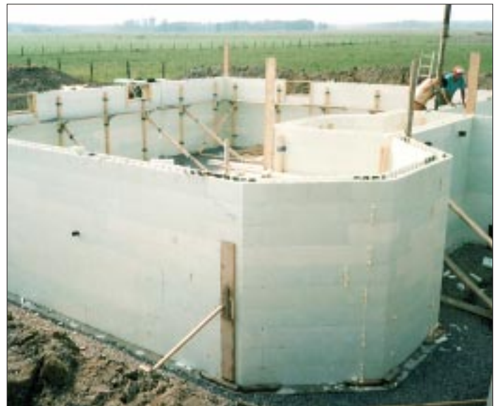
Figure 3. Large-core molds use less concrete than block or sheet forms. Large horizontal and vertical cores, reinforced and filled, produce a post-and-beam structure.
