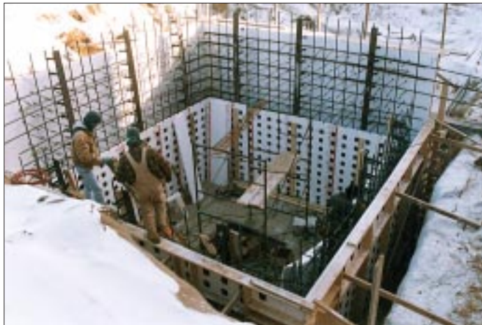
Figure 2. Sheet forms, like R-Forms (top) and Lite-Forms (above), assemble and fill like conventional plywood forms.
