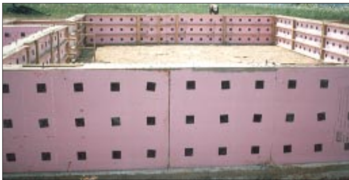
Figure 1. Some stackable blocks, like SmartBlocks (top), snap together like Legos; others, like the Ice Block (above), use a tongue and groove.
