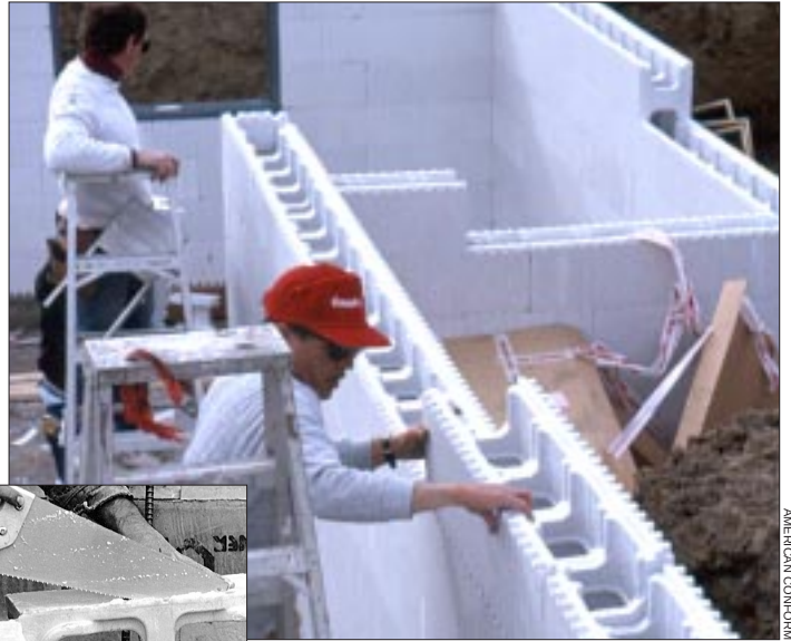
Though they don't save money, stackable foam blocks form and insulate in one step. They are lightweight and cut with a handsaw (inset).
