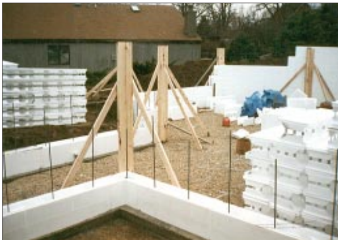
Figure 1. Some stackable blocks, like SmartBlocks (top), snap together like Legos; others, like the Ice Block (above), use a tongue and groove.
