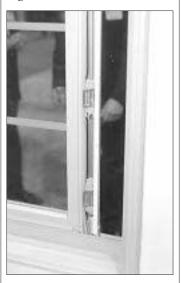
Today's windows lose more heat through air leakage between the sash and the jamb than by conduction through the glass and frame. Air leakage is measured in cubic feet per minute per linear foot of crack (cfm/ft.) with a 25-mph wind blowing directly at the window. Casement and awning windows are pretty tight (testing as low as .01 cfm/ft.), but gliders and doublehungs are a lot draftier.
