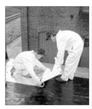
Here's a way to cover a low-slope roof without getting tar on your pants. *Peel and Seal*, a self-stick roll roofing, is a 45-mil membrane that consists of an aluminum foil surface, a thin polymer film, and a thicker substrate of rubberized asphalt. It's designed for use on free-draining roofs (ones with no ponding water) with a minimum slope of 1/2 inch per foot.
