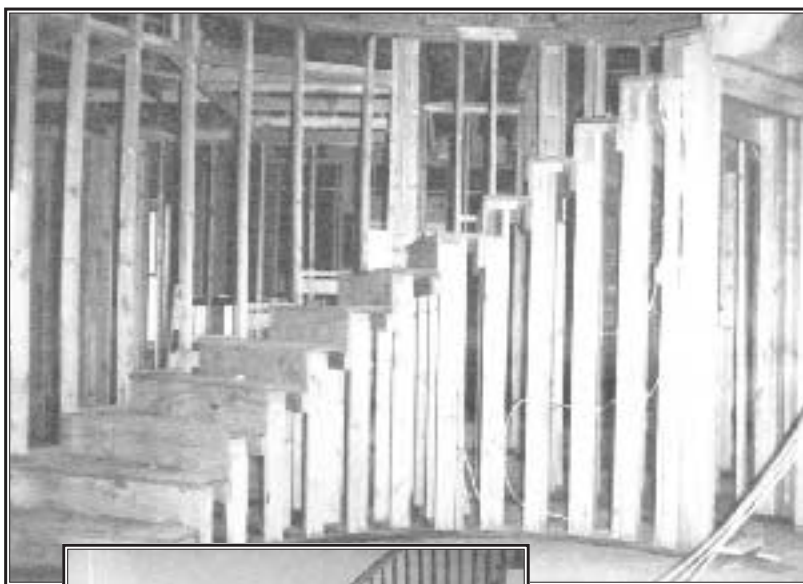
This elegant curved stair conceals a frame structure (above) consisting of a series of stepped walls fanned out along an arc and tied together by plywood treads and risers.
