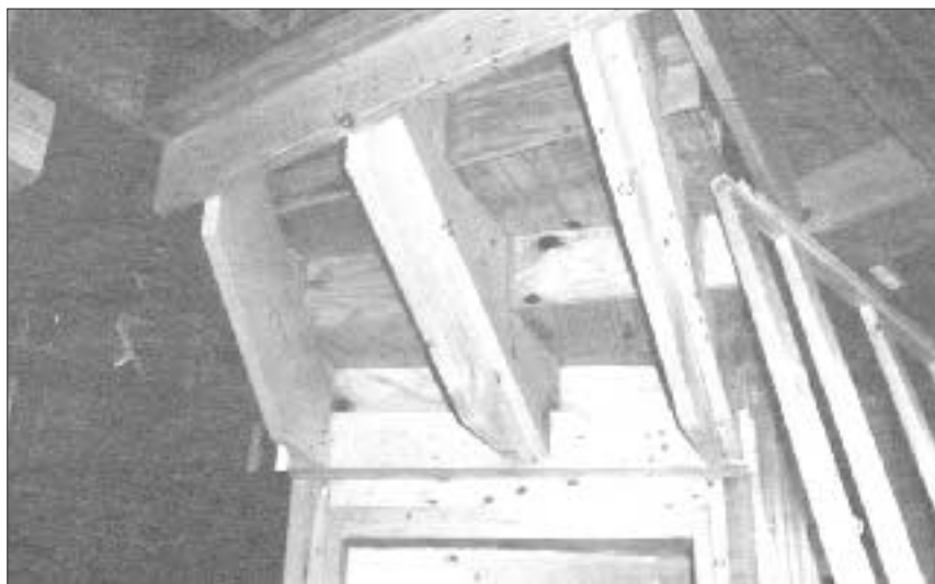
Figure 2. Simple pony walls, framed 16 inches on-center, support the first eight treads of the stair. The next five pony walls include a header to span the closet opening. A 2x ledger fastened 6 1/8 inches below the top of each wall supports the back of each tread.
