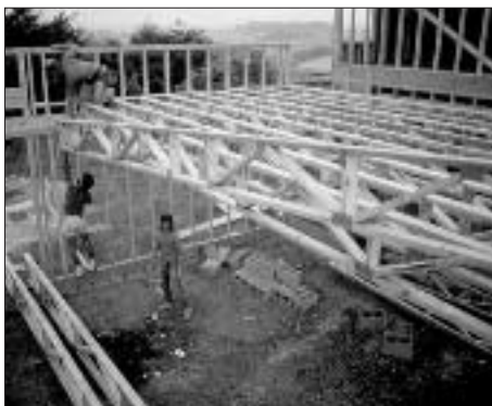
Figure 3. Floor trusses are usually lifted into place by hand (left), though fork lifts and cranes can speed the process (right).
