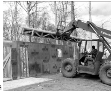
Figure 3. Floor trusses are usually lifted into place by hand (left), though fork lifts and cranes can speed the process (right).
