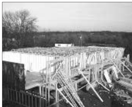
Figure 2. The job foreman on this multi-family building estimated that the floor framing took half as long with trusses as it would have with standard dimensional lumber.
