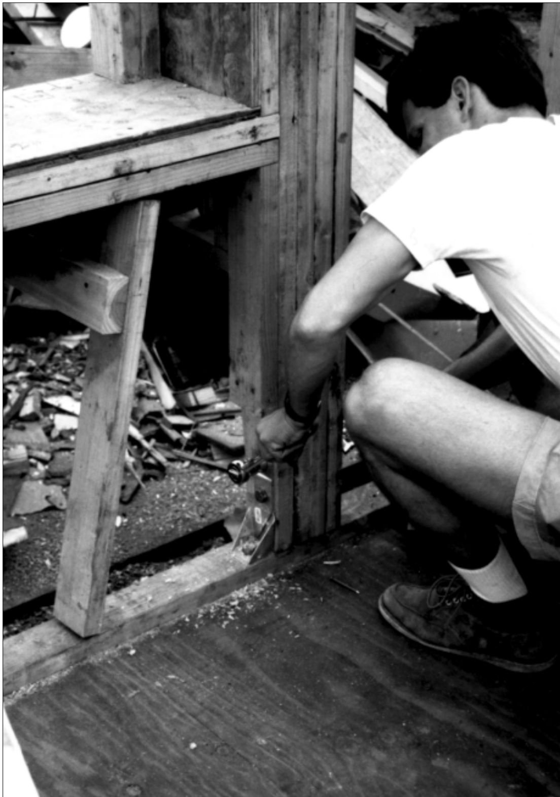
Carpenter Craig Lauchner of Mountain View, Calif., cinches down a nut on a foundation hold-down at a bay window opening. A cripple stud has been temporarily pushed aside to make room for drilling the bolt holes in the framing.
