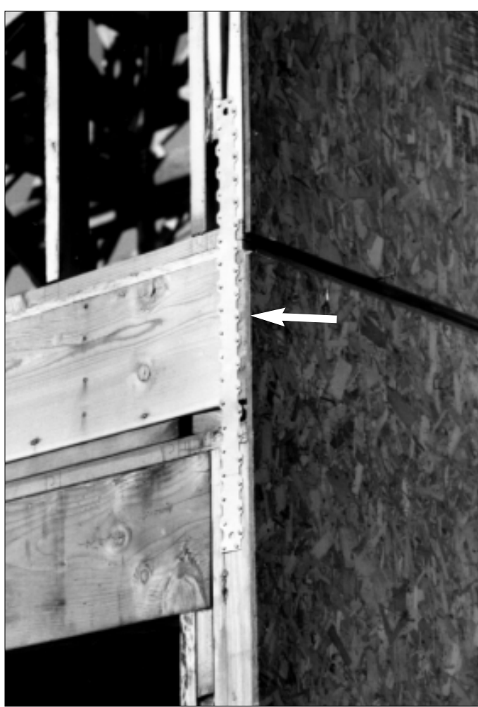
Figure 7. Wall connectors come in two varieties. You can use hold-downs bolted together through the floor assembly (left) or nail strap ties into the studs (right).
