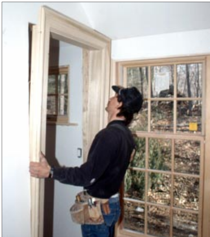
A carpenter installs an interior door precast with custom moldings.
