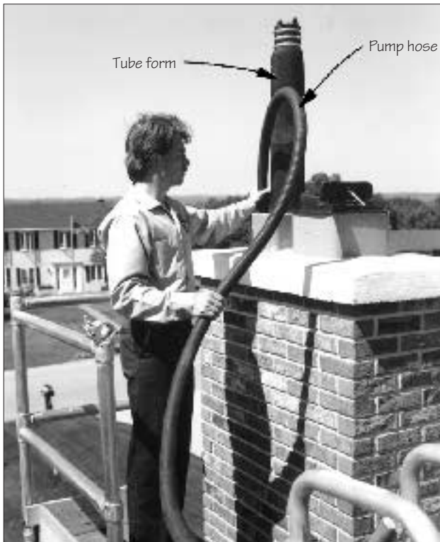
Figure 4. Cast liner installation. Starting with an unlined chimney (A), a rubber tube form is inflated with air, then centered between the chimney walls. Next, the liner material is mixed and pumped into the chimney (B). After the mix sets up, the tube is deflated and removed, creating a flue (C). Depending on the fuel to be burned by the appliance, the flue may have to be sealed.
