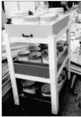
Figure 2. This site-built cart organizes a variety of one-gallon buckets that hold the metal hardware frequently needed on remodeling jobs.
