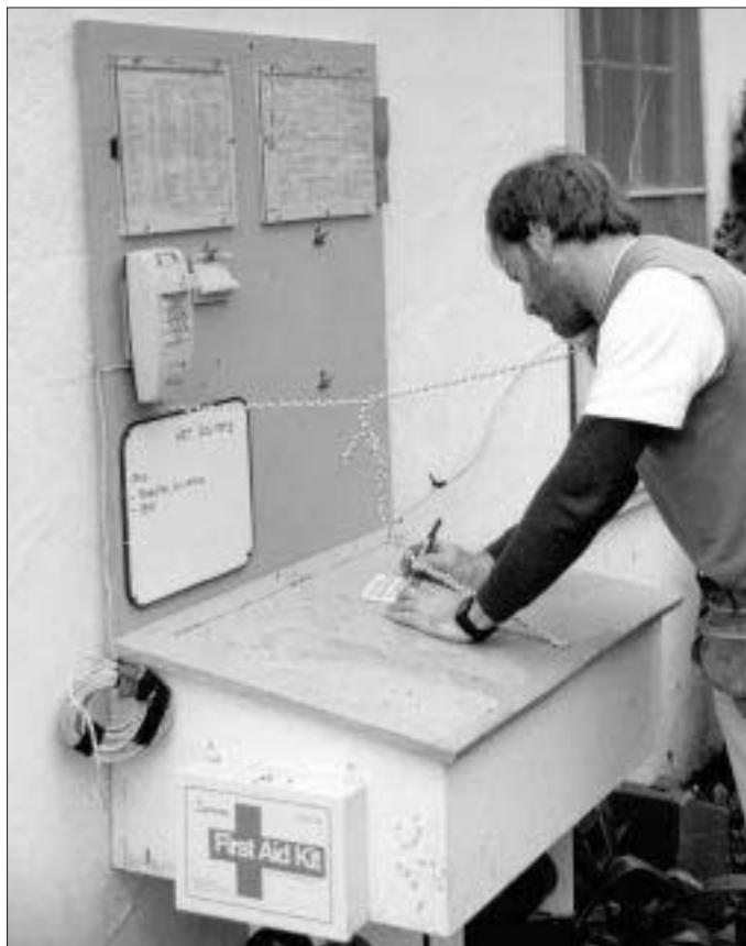
This portable telephone desk mounts easily to a framed wall, providing a convenient location for plans, telephone directory, inspection card, and messages for the client. The storage area under the desk top holds small parts that can be easily lost during the course of a job. An outlet box inside is for cordless battery chargers.
