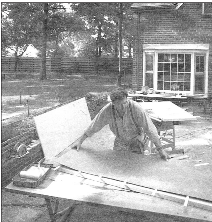
Figure 5. Place stickers 12 inches on-center to keep the surface laminate from adhering to the substrate as it is being positioned.
