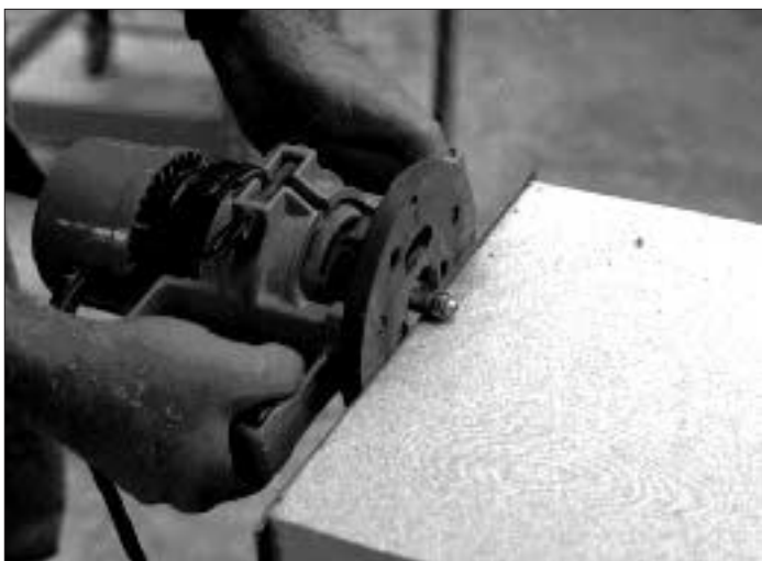
Figure 4. Apply and trim laminate edges first, beginning with the ends of the countertop.
