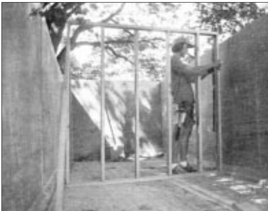
Figure 3. Instead of buying or renting a different container for each type of recyclable material, you can build a partition inside a standard dumpster to segregate your waste.
